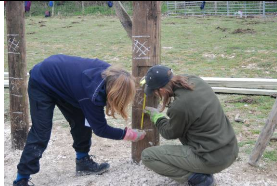
Rail positions are marked on the posts.
