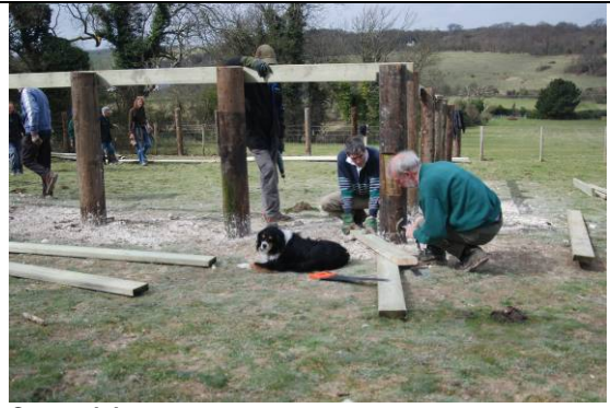
Corner joints are cut...
