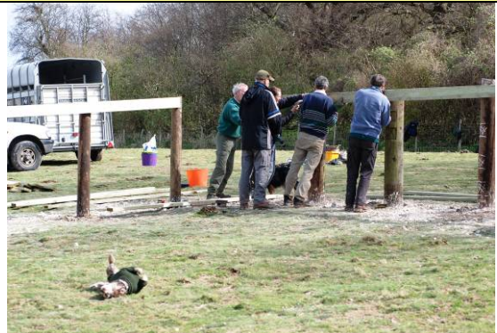
The top rails are levelled and nailed in place, while Assistant Warden "Res" finds something interesting to roll in.
