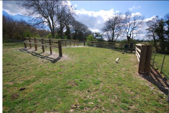
Fencing complete – delivery of gates delayed.
